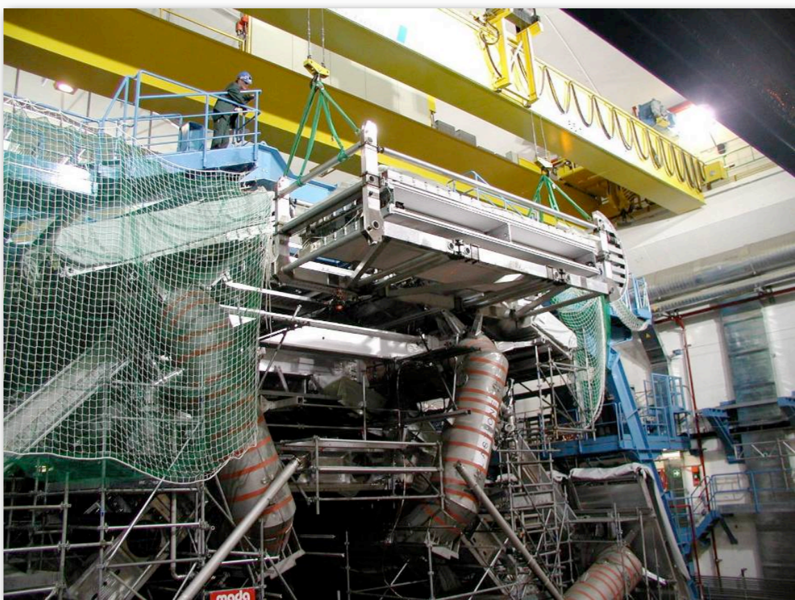
Installation of barrel muon chambers (~700) started in Nov 2005 and is ~ completed
