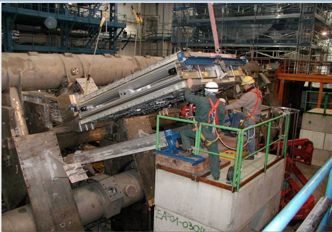
Installation of barrel muon chambers (~700) started in Nov 2005 and is ~ completed
